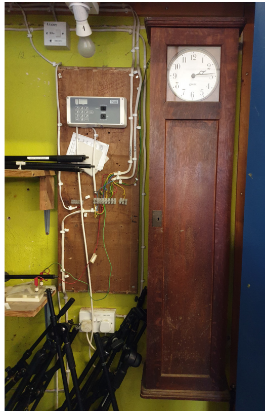
Fig. 4. Gent C7 impulse transmitter, No. 4955 (29 August 1938), now a rather forlorn relic in a cupboard in the corner of the Green Room. Photo Sue Hines.
