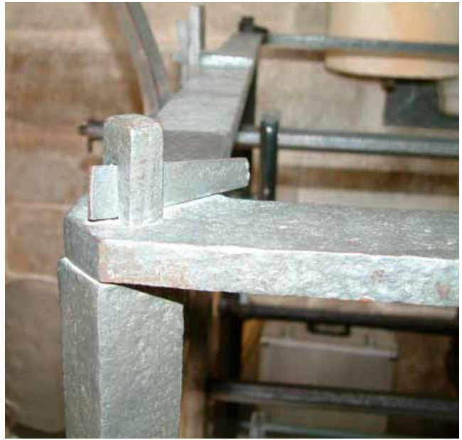
Fig. 18. Detail of the top corners of Salisbury and Wells. Both are constructed in the same manner.
