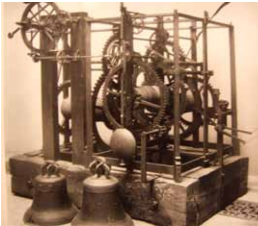
Fig. 2a. The Wells clock in an old photograph.
